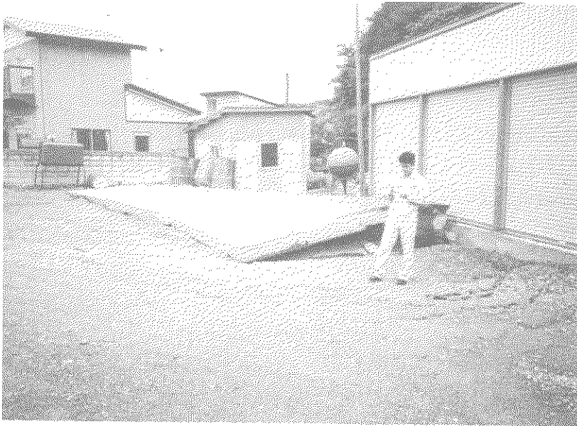
Photo 6 Built-up the Oil pit due to Liquefaction
